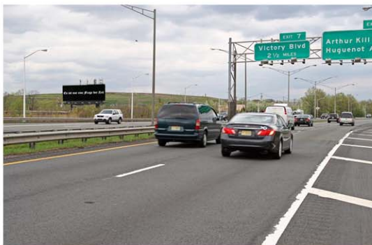
Westshore Expressway/Route 440, south of Arden Ave, Staten Island, NY
